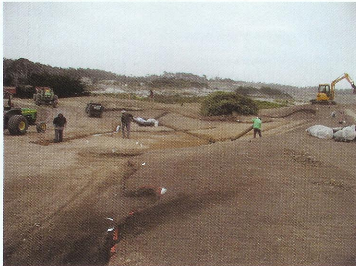
Workers install drain pipe and sand capping to resolve chronic drainage problems at Monterey Peninsula Country Club Shores.
